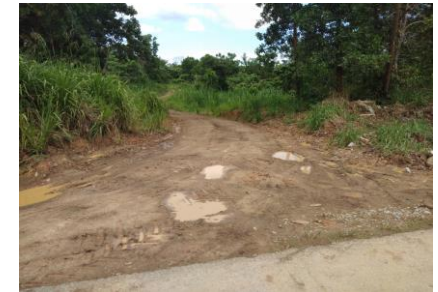
Earth road inside project site
